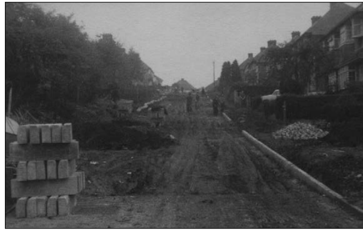
Geralds Road under construction in the early 1930s. (Jean Finlan collection)
