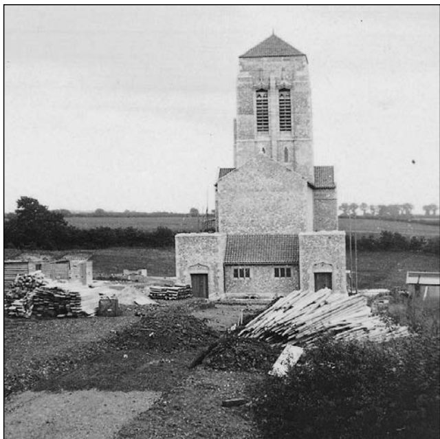
St Francis' Church nearing completion, 1930. (Len Owen)
